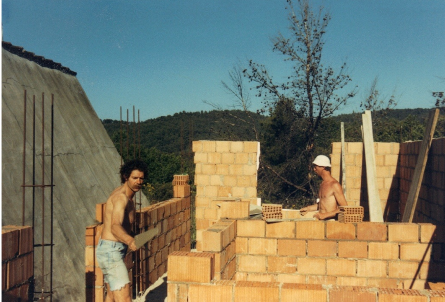
Jacques & I building the extension.
